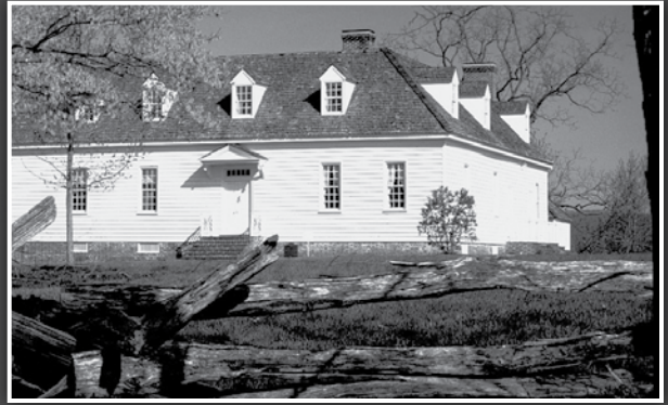
Col. William B. Preston established the Smithfield estate – named for his wife, Susanna Smith – in 1772 after an earlier settlement known as Draper’s Meadow was wiped out in an Indian massacre. The oldest part of the existing house was built in 1790. A state historic landmark, Smithfield is open for tours April through November. Call (540) 951-2060 for details.
