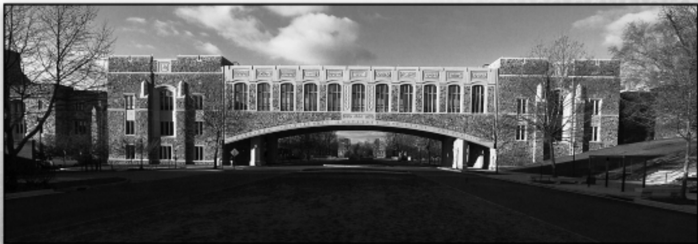
Torgersen Hall, home to Virginia Tech's Advanced Communications and Information Technology Center, provides a high-tech environment in which researchers, teachers and students can interact in innovative and effective ways. The building includes high-tech auditoriums; observational booths for watching and taping experimental teaching techniques; the CAVE, Tech's sophisticated virtual reality environment for advanced research and learning; and an electronic reading room occupying the arch that spans the Mall.
