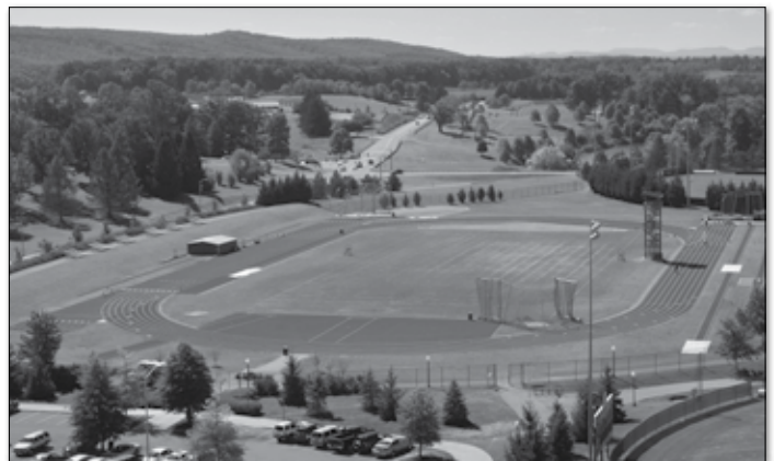
The outdoor oval track at the Johnson-Miller Outdoor Track Complex has eight 42-inch lanes and is identical to the track used in Atlanta's Olympic games.
