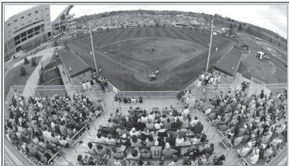
With permanent seat-back bleachers, handicap accessibility and a modern press box, Tech Softball Park (above) has become one of the best facilities around and always draws great crowds to Hokie softball games (below). Last year, Tech averaged 551 fans per contest, 17th-best in the nation.
