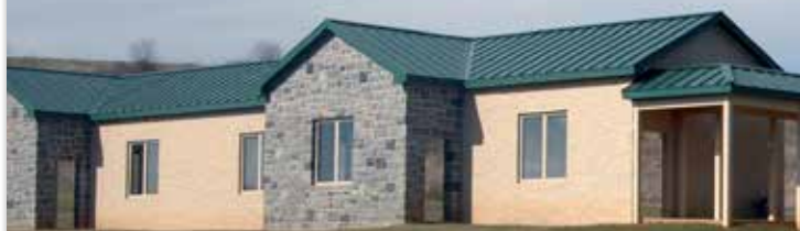
The Virginia Tech Golf Team Complex, complete with indoor and outdoor practice facilities, putting green and short-game area, at the Pete Dye River Course of Virginia Tech.
