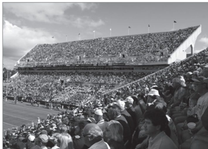
The South End Zone is an imposing structure for opposing teams.
