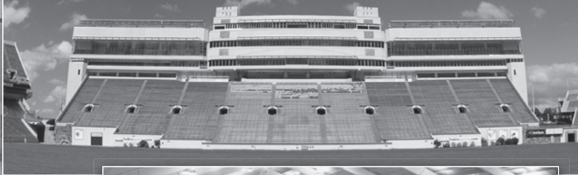
The west side expansion of Lane Stadium is a magnificent new structure.
